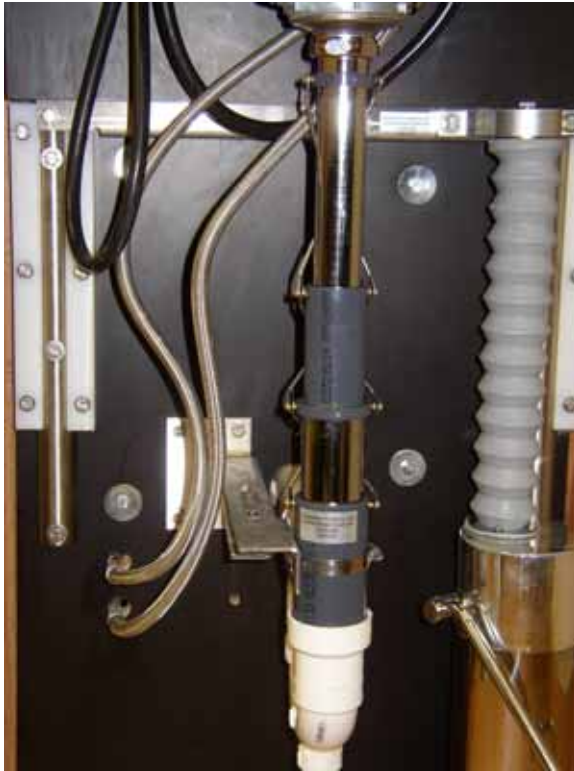
Note: The lift system limits out prior to the drain limiting out, the drain is perpendicular to the floor, and the cables face the wall
